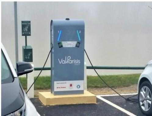
Figure 7 - Borne CITY (2x22 kW) – TOTAL EV CHARGE
