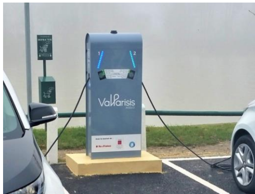
Figure 7 - Borne CITY (2x22 kW) – TOTAL EV CHARGE
